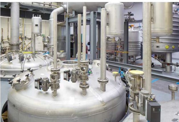
Two reactors for the adhesive polymerization under construction, the control fittings (ball sector valves) have already been mounted on the supply lines.
